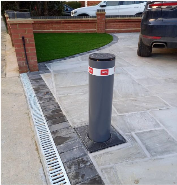
RJL automatic bollard installation. Note the strip drain at the bollard.
